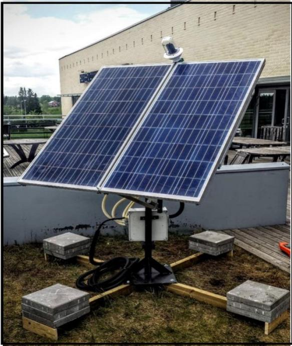
Figure 6: dual-axis solar tracker
