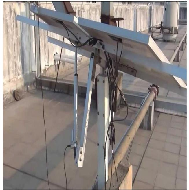
Figure 8: dual-axis solar tracker
